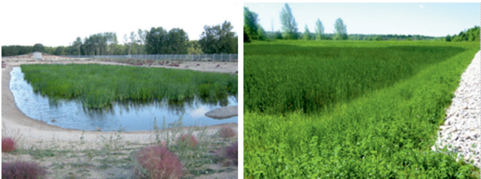
Fig. 46. Examples of free-water system (FWS) (left) and subsurface flow system (SFS) (right) wetlands
