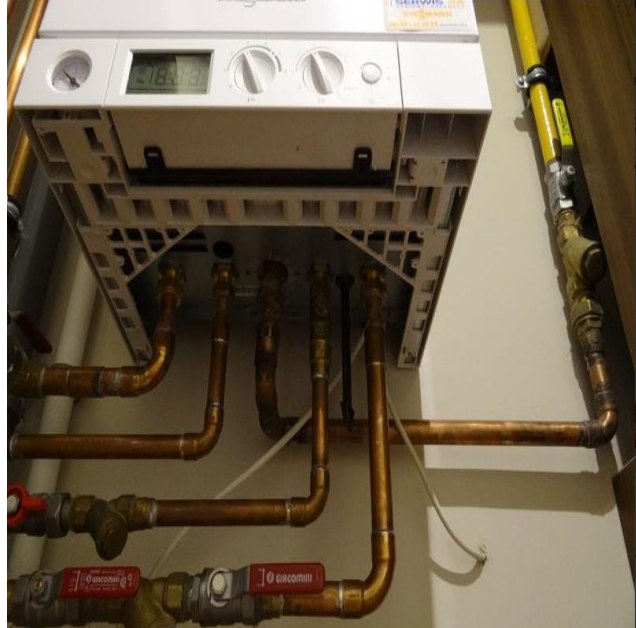
Bringing the installation to a dual-function gas boiler
