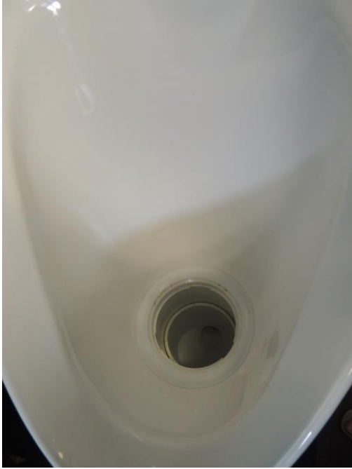
The pictures present an example of a trap for waterless urinals.
