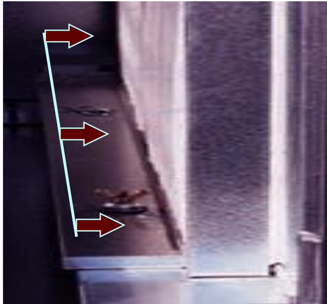
Pressure mounting of pre – filters
